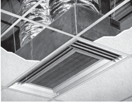
LIGHT COMMERCIAL "T" BAR CEILING
