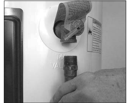
Figure 13 - Removing the T&P Relief Valve discharge pipe.
