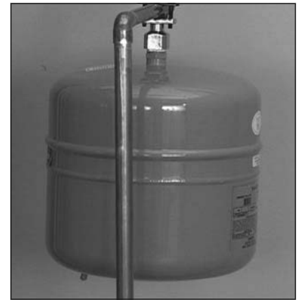
Figure 7 - A Thermal Expansion Tank helps protect the home's plumbing system from pressure spikes.
