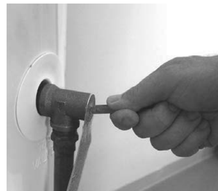
Figure 46 - T&P Relief Valve
