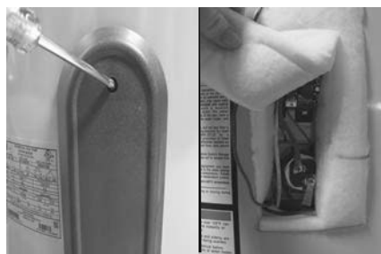
Figure 45 - Element Access Panel/ECO Compartment
